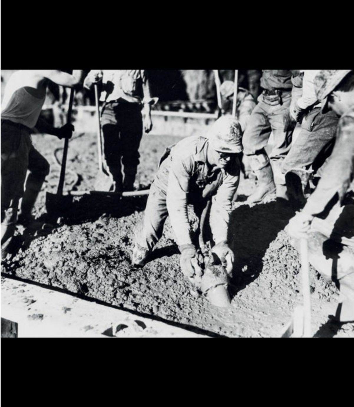
Workers compact concrete used to build the Boulder Dam (later renamed the Hoover Dam), located on the border of Arizona and Nevada, 1934. Kahn's multiplier suggested that each dollar spent on a public works project like this would boost national output by more than one dollar.
