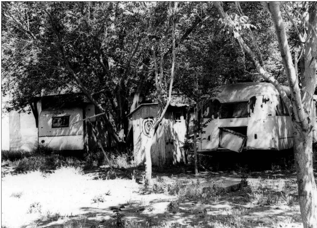
Trailer trash as squatters in Arizona (1950).
